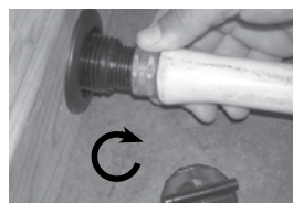
3. Thread hose onto the spa drain
